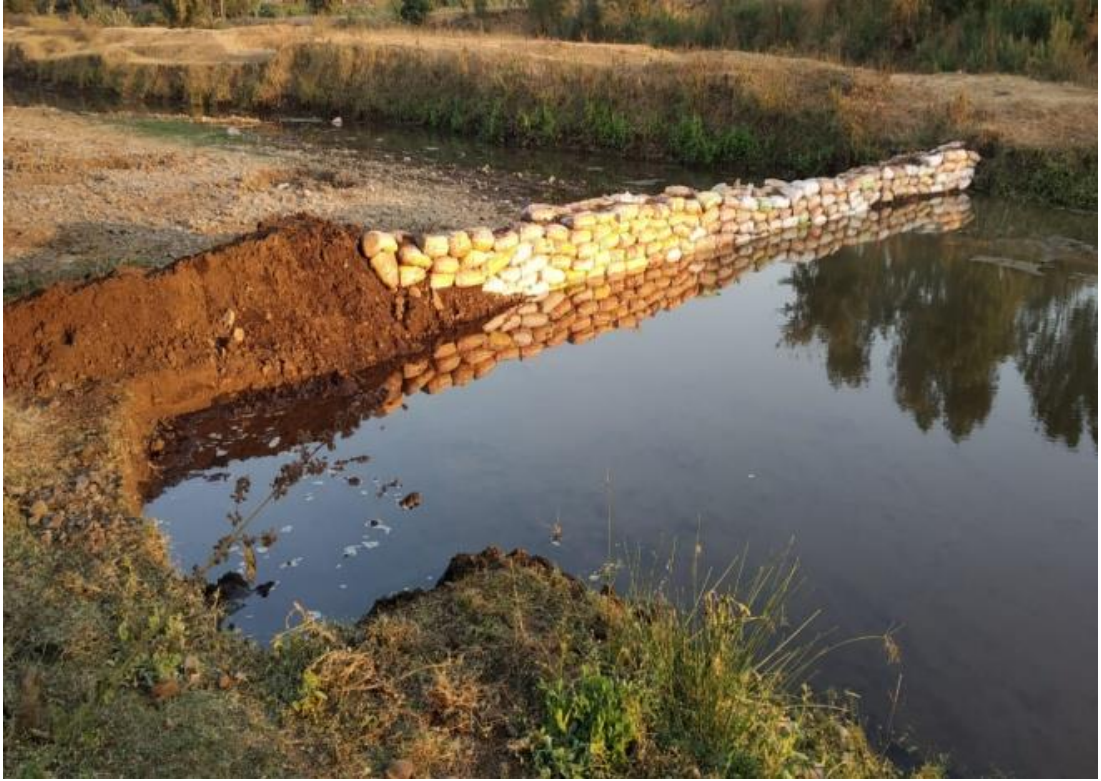
Vanrai dam No. 1
