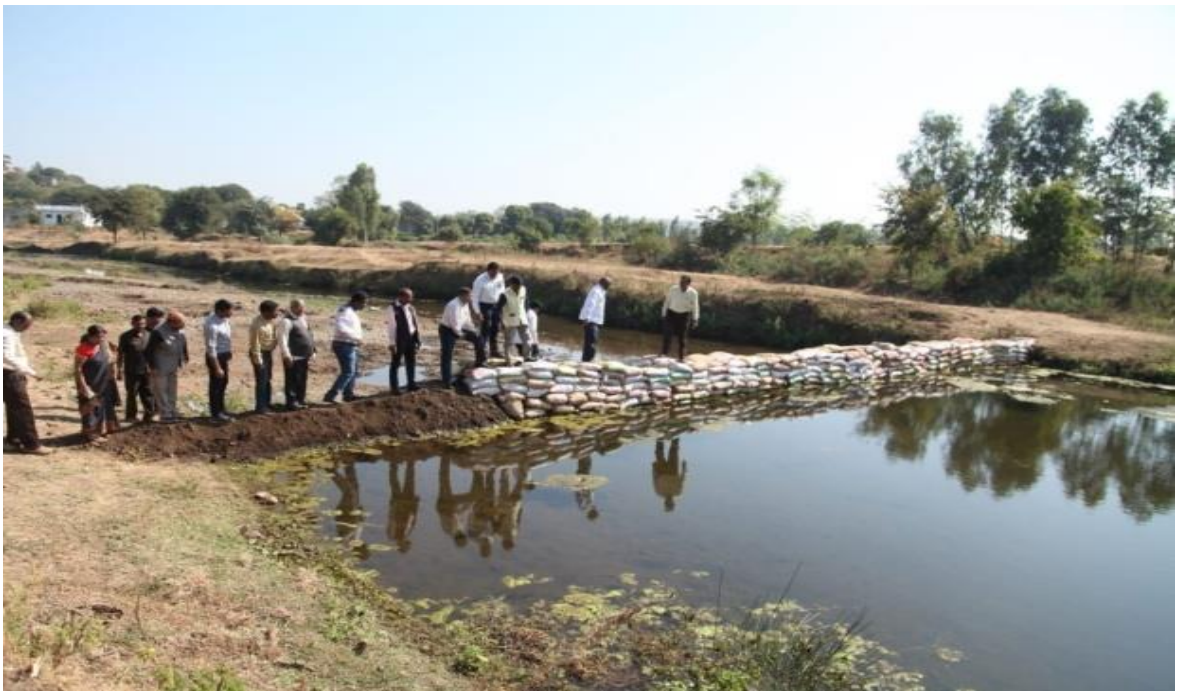
Vanrai dam No.8
