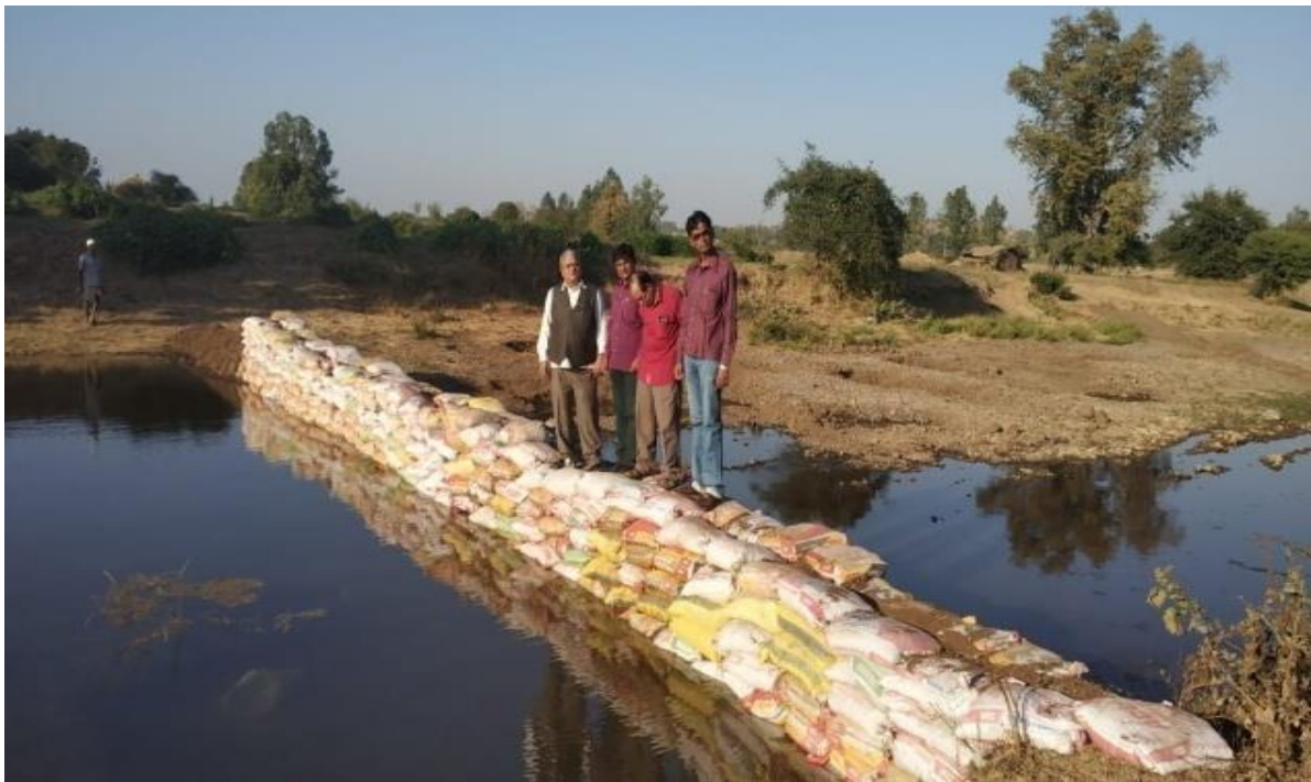
Vanrai dam No.6
