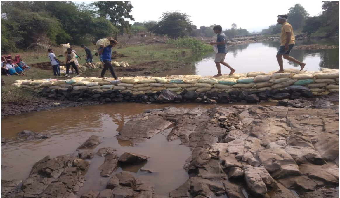
Vanrai dam No.11
