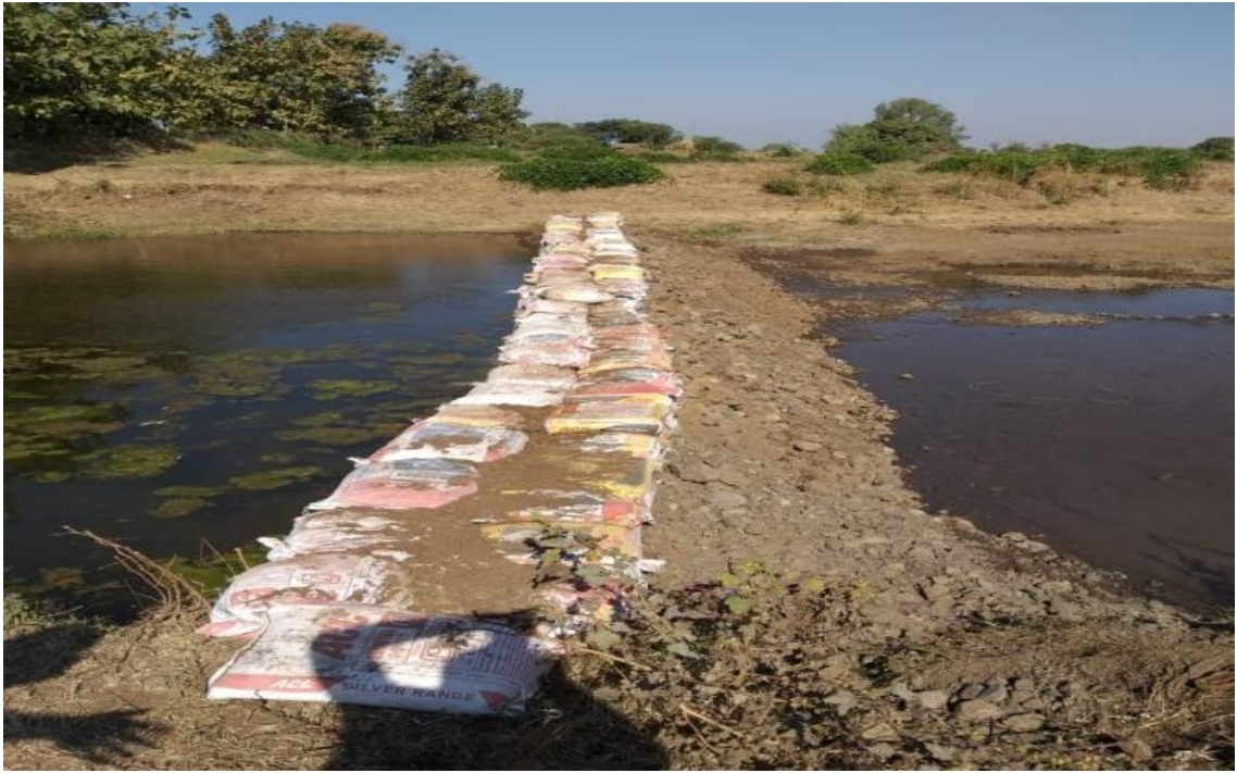
Vanrai dam No.3
