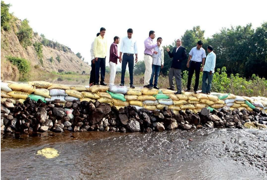
Vanrai dam No.5
