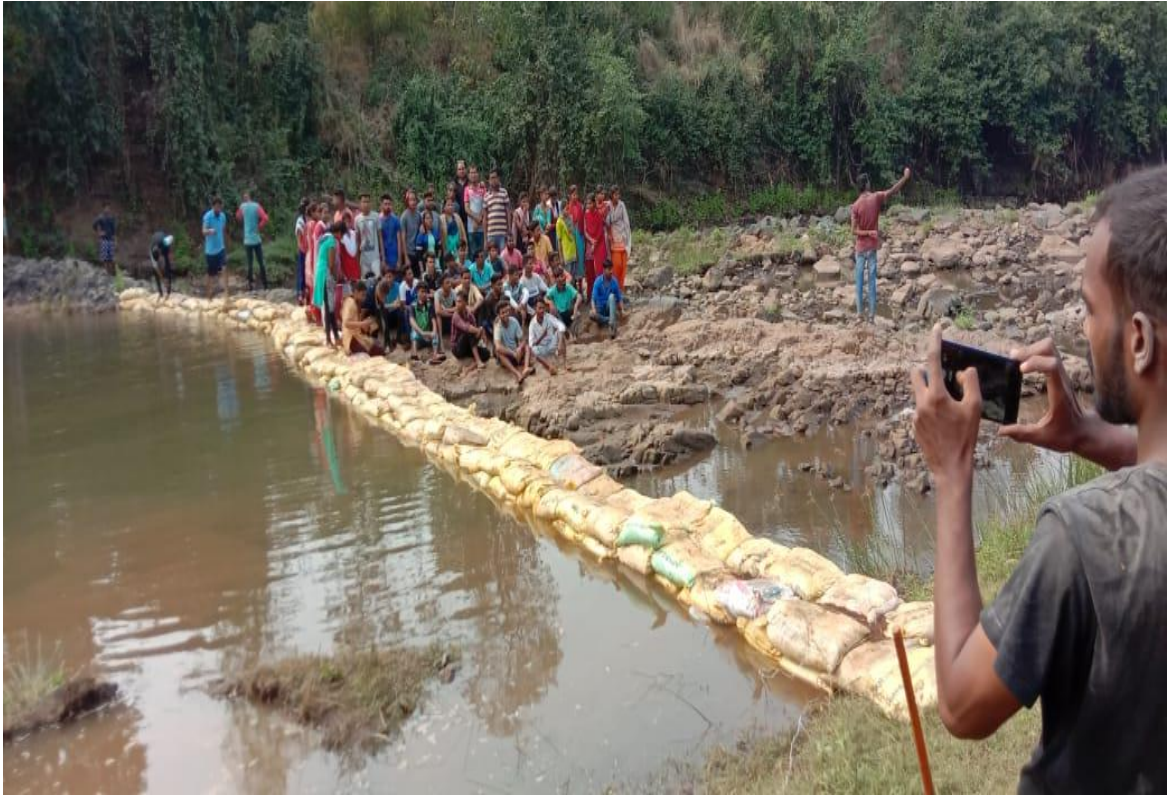
Vanrai dam No.12
