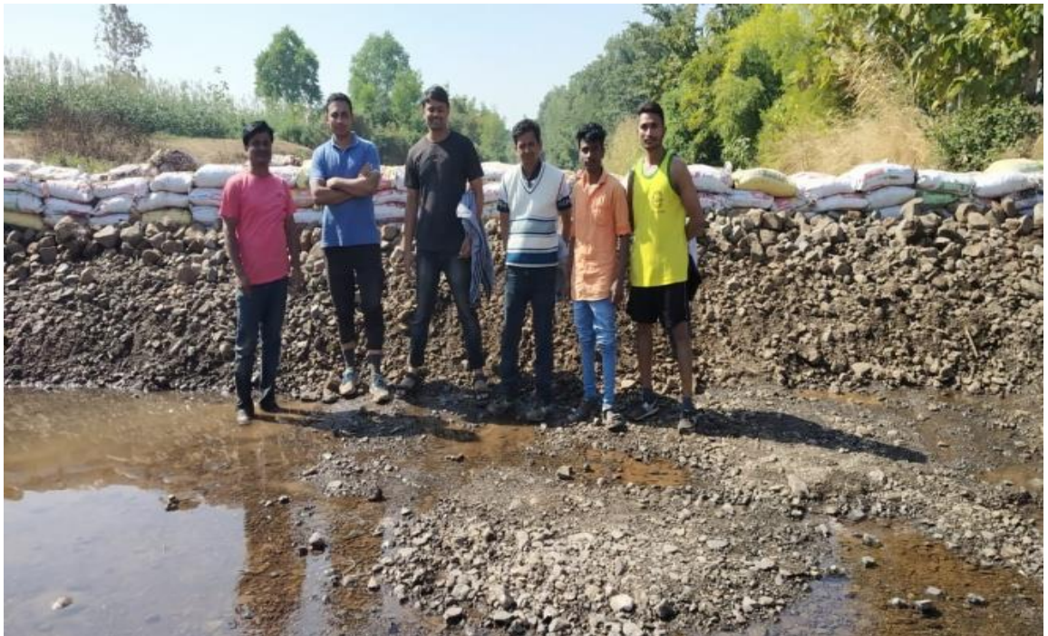
Vanrai dam No.2
