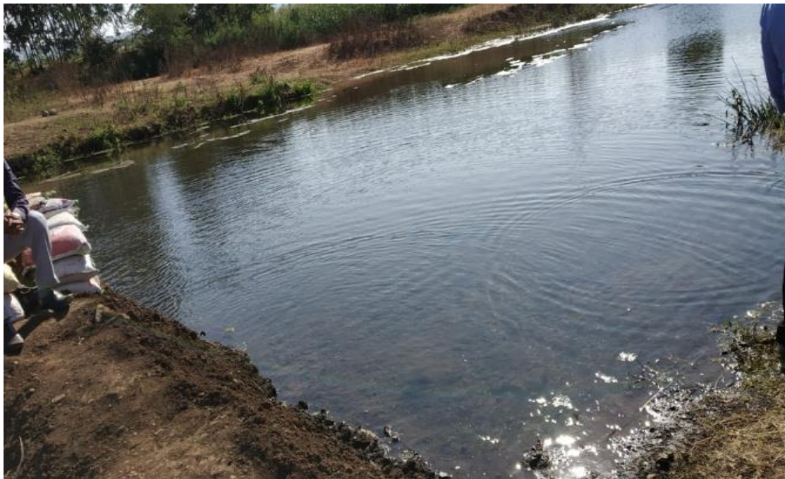
Vanrai dam No.4
