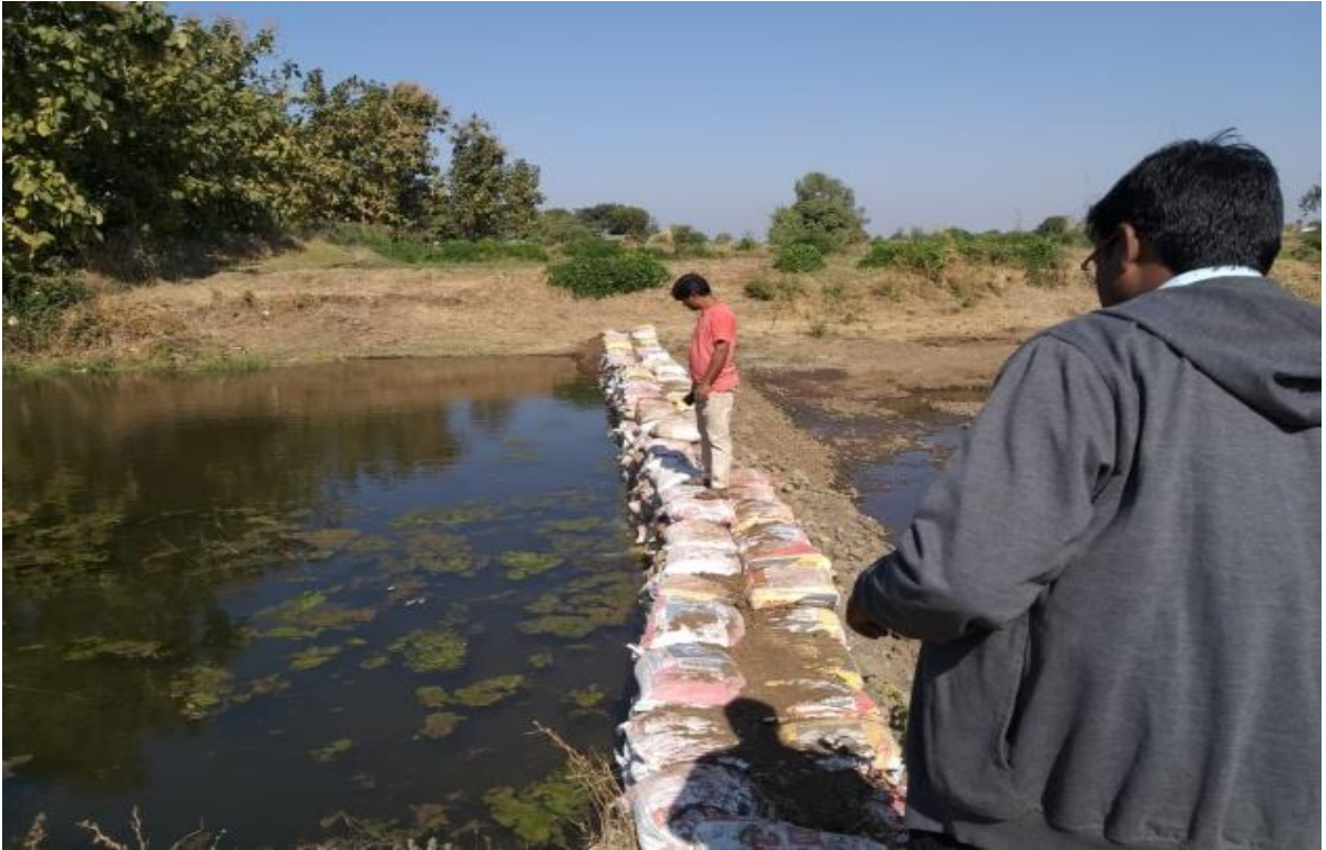
Vanrai dam No.7
