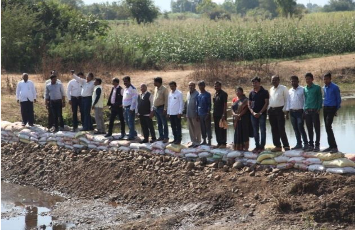
Vanrai dam No.9
