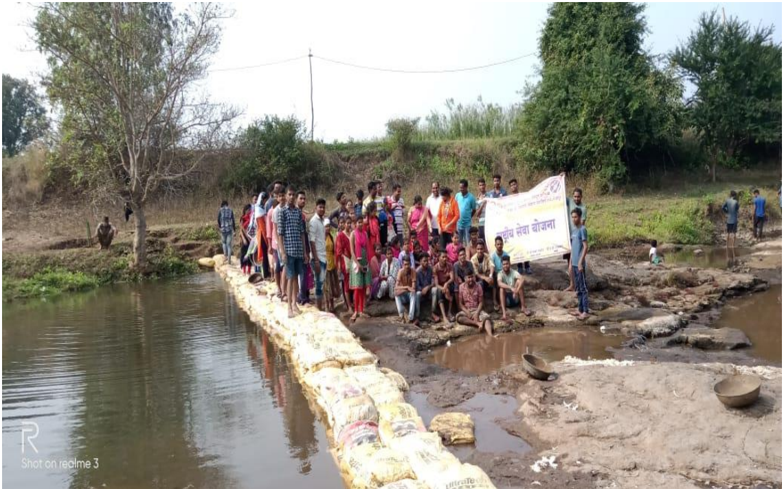
Vanrai dam No.13
