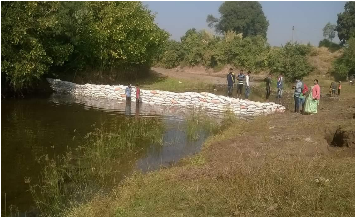
Vanrai dam No.10
